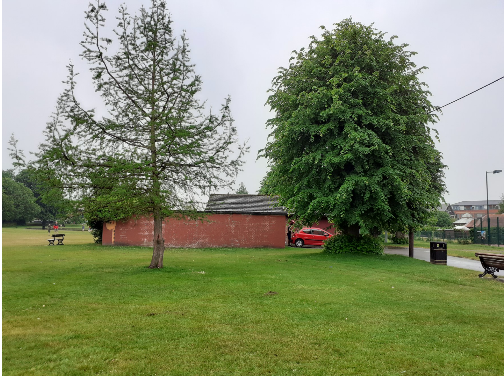
North elevation of storage building and kiosk
